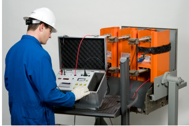
Figure 8: FMFC Applied around Entire Pole
